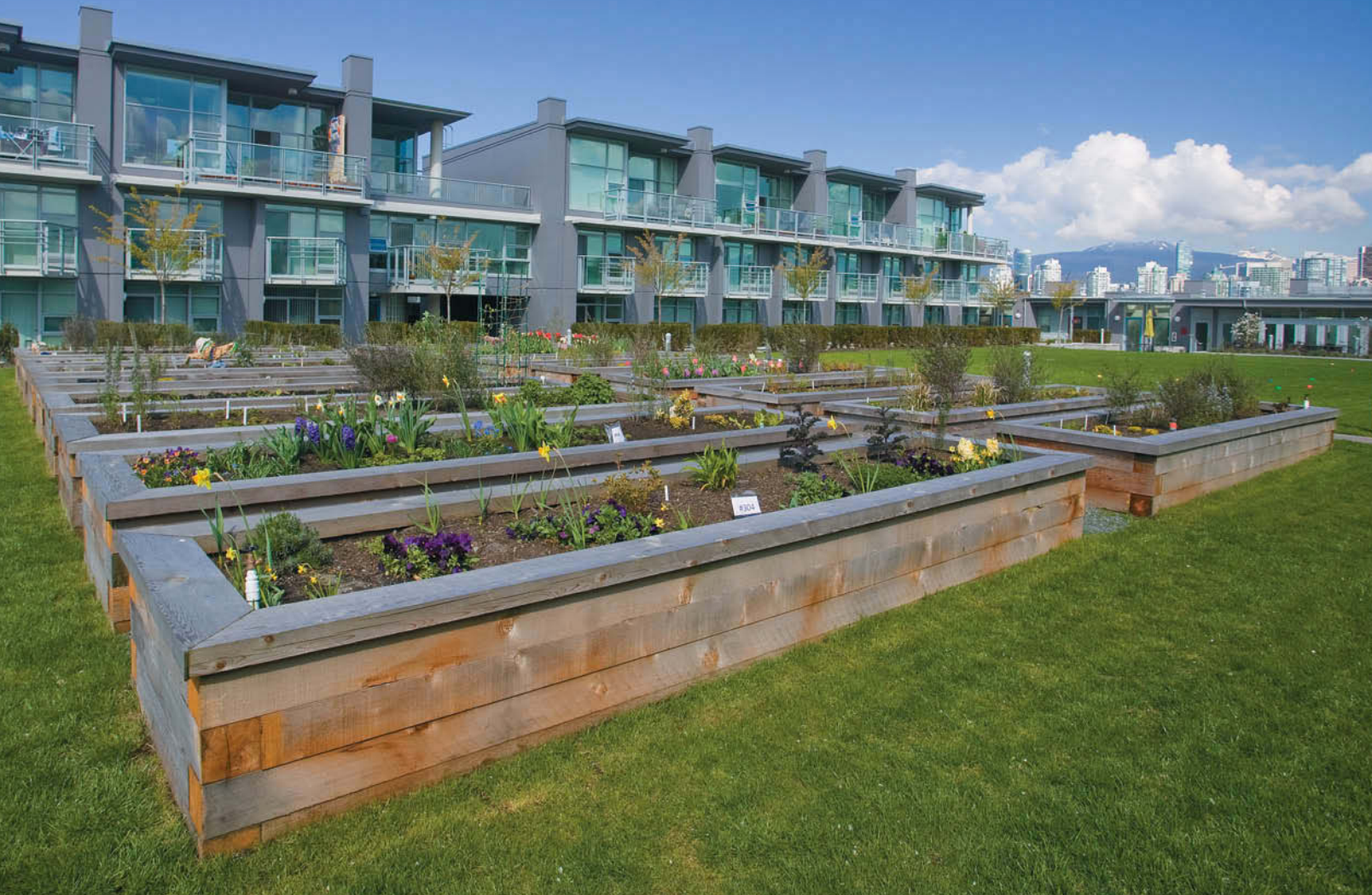
Rooftop garden with raised planter boxes at The Rise, an award-winning mixed-use infill development in Vancouver.
